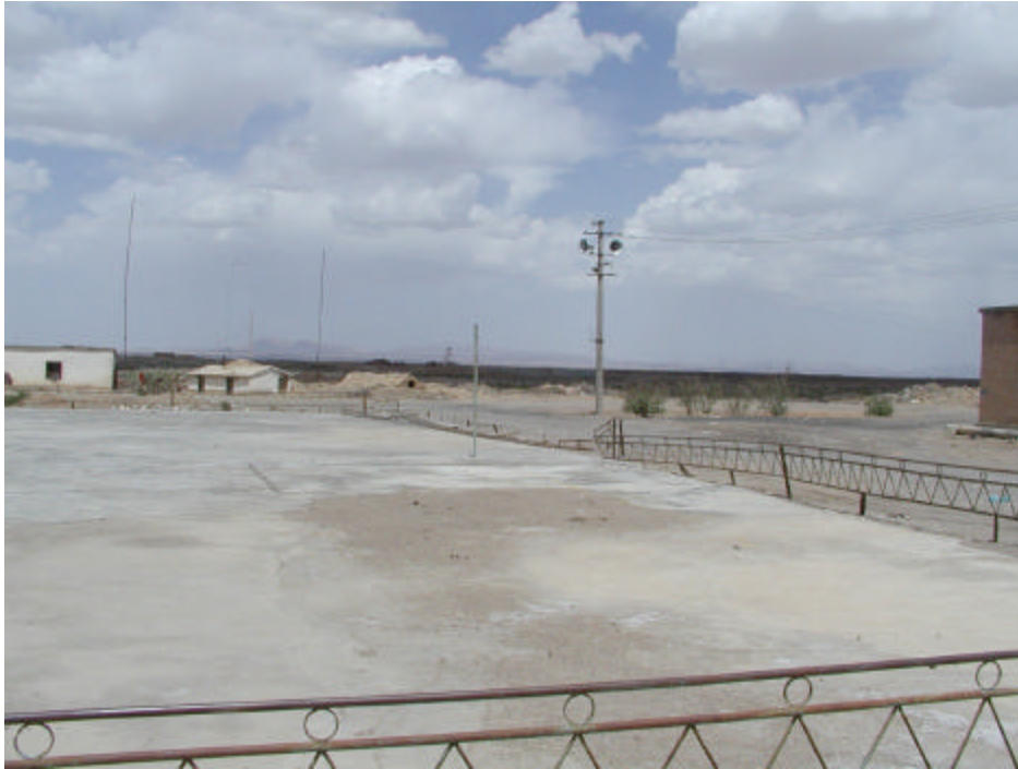
Photo HM-1: Xinwozi Mine area building.
