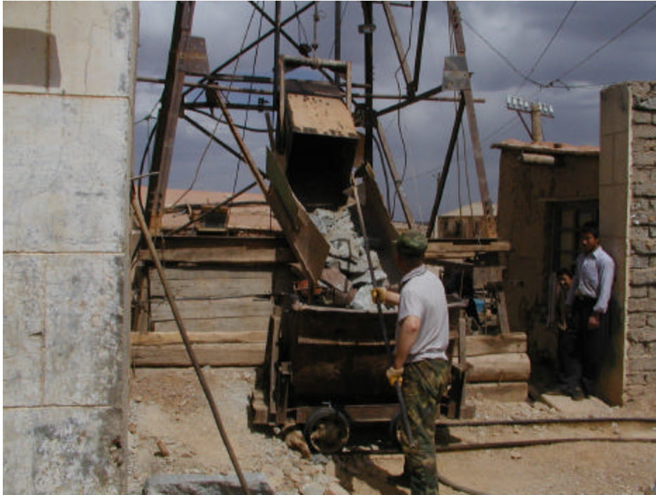
Photo HM-11: Loading ore car at Quartz Vein #49 shaft.
