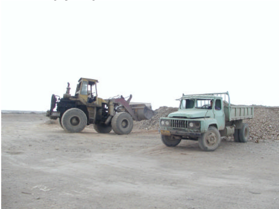
Photo HM-18: Loading operating at 210 Zone.
